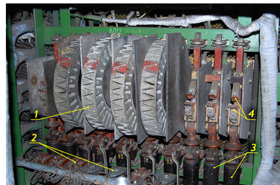
Powerful DC contactor with electro-pneumatic drive
