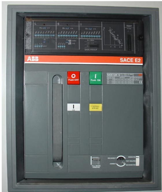
Front panel of a 1250 A air circuit breaker manufactured by ABB. This low voltage power circuit breaker can be withdrawn from its housing for servicing. Trip characteristics are configurable via DIP switches on the front panel.
