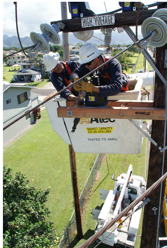
Working on high voltage power lines
