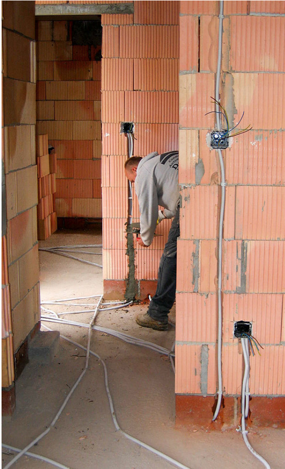
Installing electrical wiring by cutting into the bricks of the building
